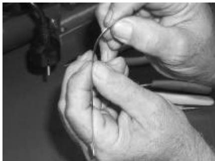
STEP A Pre-bend strap for ease of installation
